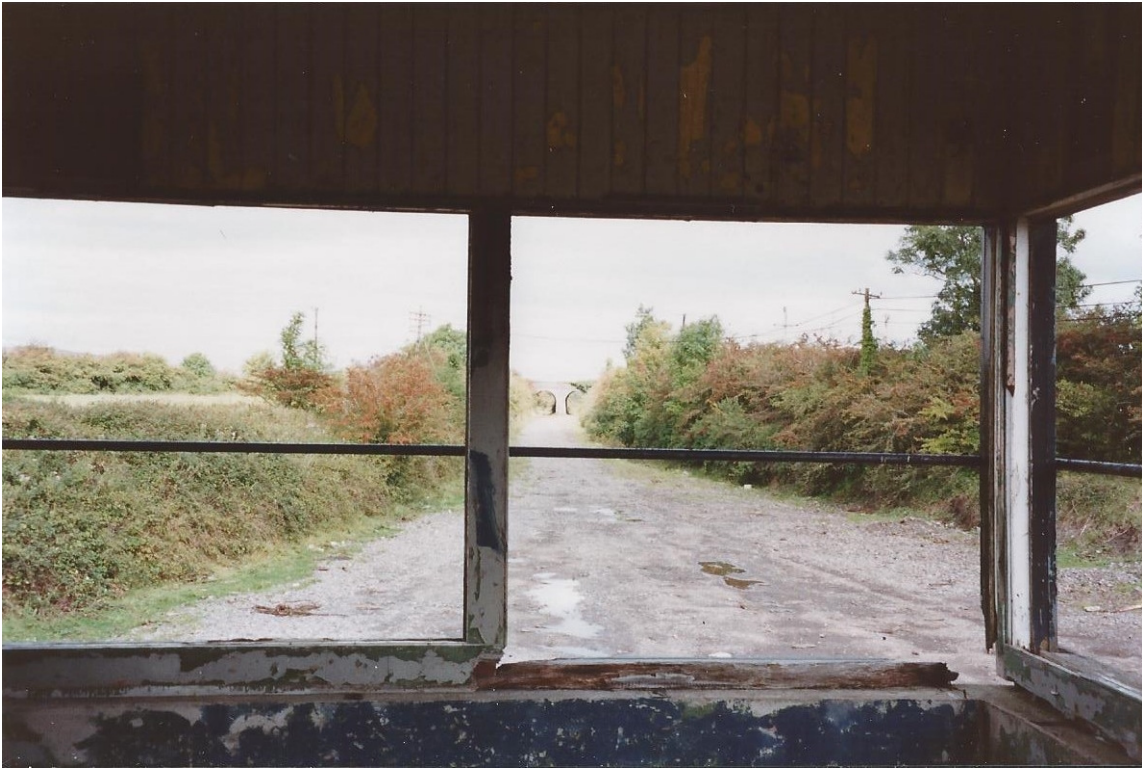
Similar view from inside the former signal cabin at Newcastle West
