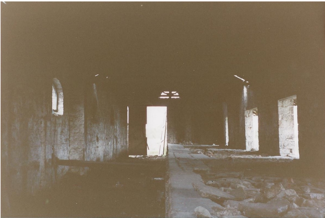
Interior of the Goods Shed at Newcastle West
